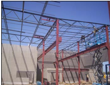
Municipal Services Building Construction
