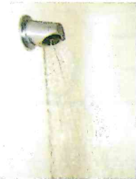
New low flow shower heads can still provide a good shower.
