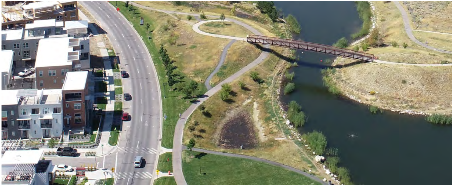
Figure 1-4: Pedestrian bridge along multi-use path in Daybreak
